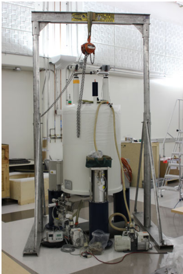
Figure 4.1: A-Frame Gantry for Lifting the Magnet Inside the Magnet Room
