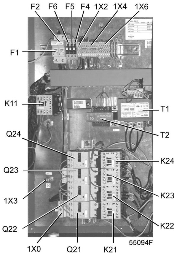
See section [Electrical diagram](#). Connect the supply cable to terminals L1, L2 and L3 of terminal strip (1X0), connect the neutral conductor to terminal (N) (if applicable) and the earthing conductor to the earthing bolt (1X3).
